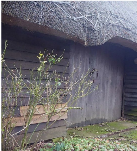
Figure 27: Weatherboarding on Bexon Manor Barn
