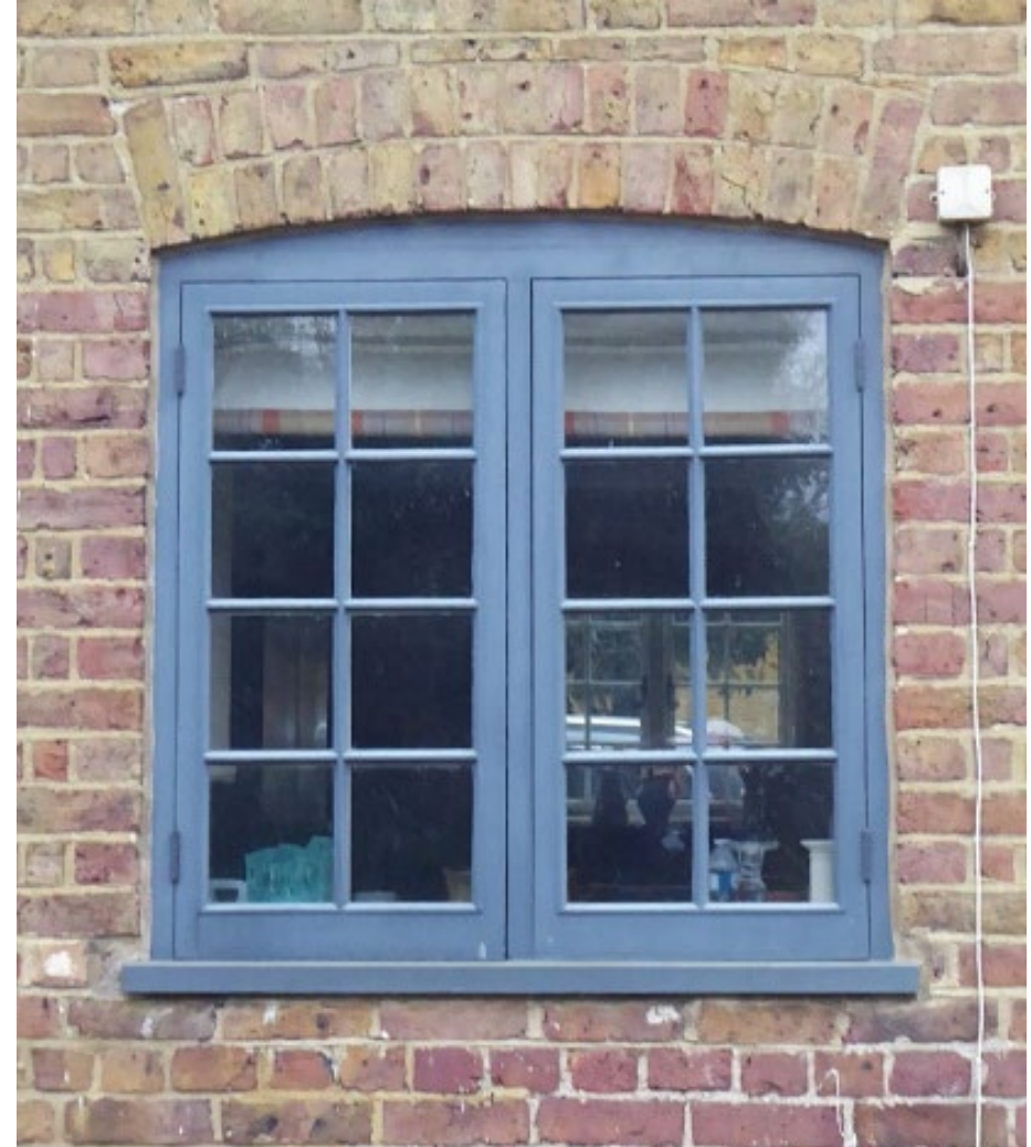
Figure 21: Modern timber window of sympathetic character at the Oast House
