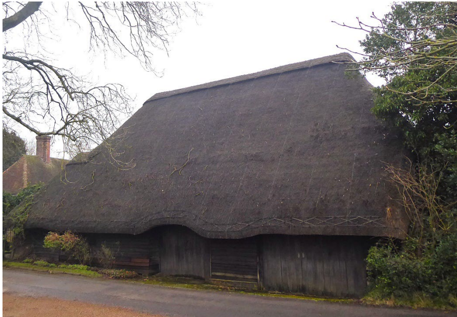
Figure 17: Barn to the south-east of Bexon Manor
