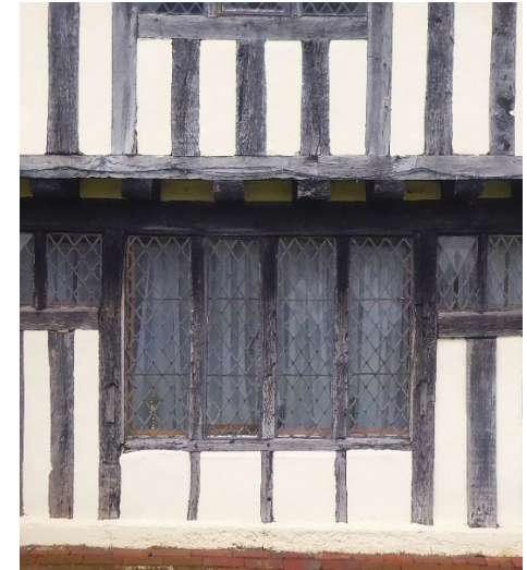
Figure 29: Historic window at Bexon Court
