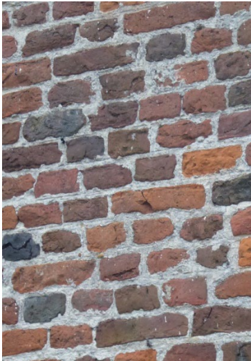
Figure 26: Early brickwork at Malt House
